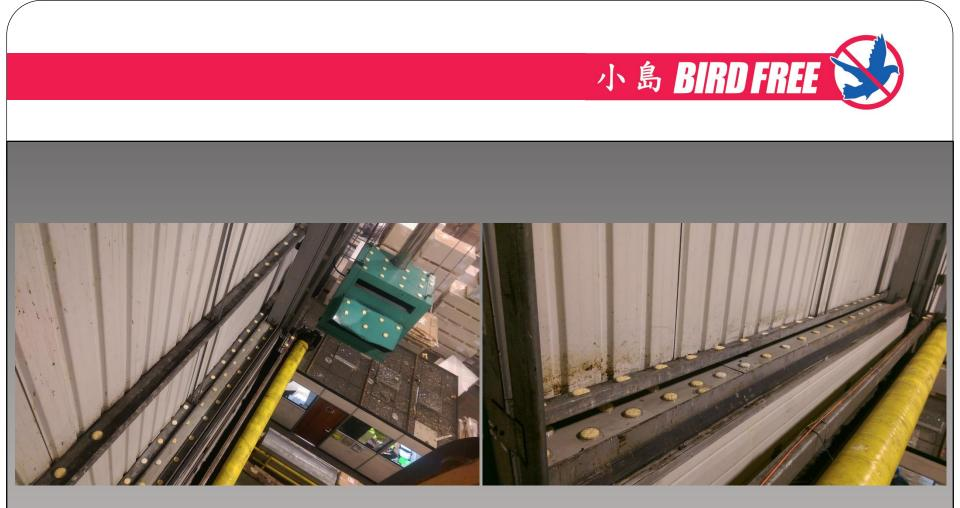
All sites from which nests had been removed were cleaned, as were the lateral beams near the nesting sites, on which the pigeons had been perching during the daytime. These were treated with 小島 *Bird Free,* as shown above.
